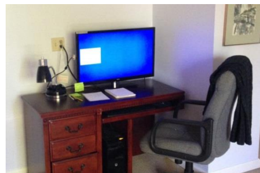
Figure 6: During this step, the project team discovered numerous lighting problems including low illumination levels, damaged cords, exposed light bulbs and this computer screen in a bedroom that was left on all night.
