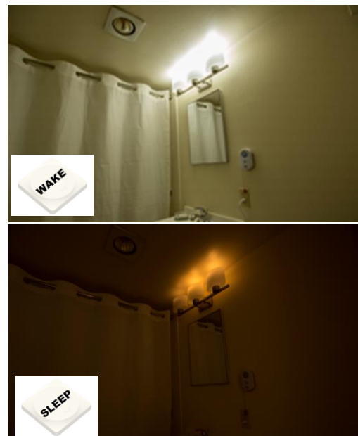
Figure 10: During waking hours, the Stack lamps were programmed to automatically change kelvin temperatures from 5000K to 2200K as shown above.
