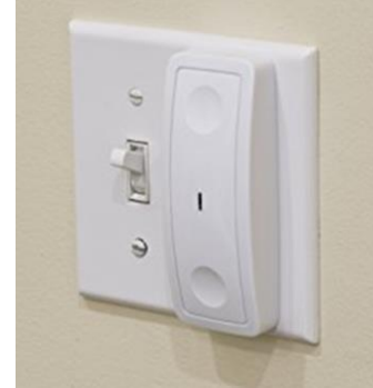
Figure 21: Since some of the residents wanted physical switches to control the lights the project team included several wireless switches like this one shown above.
